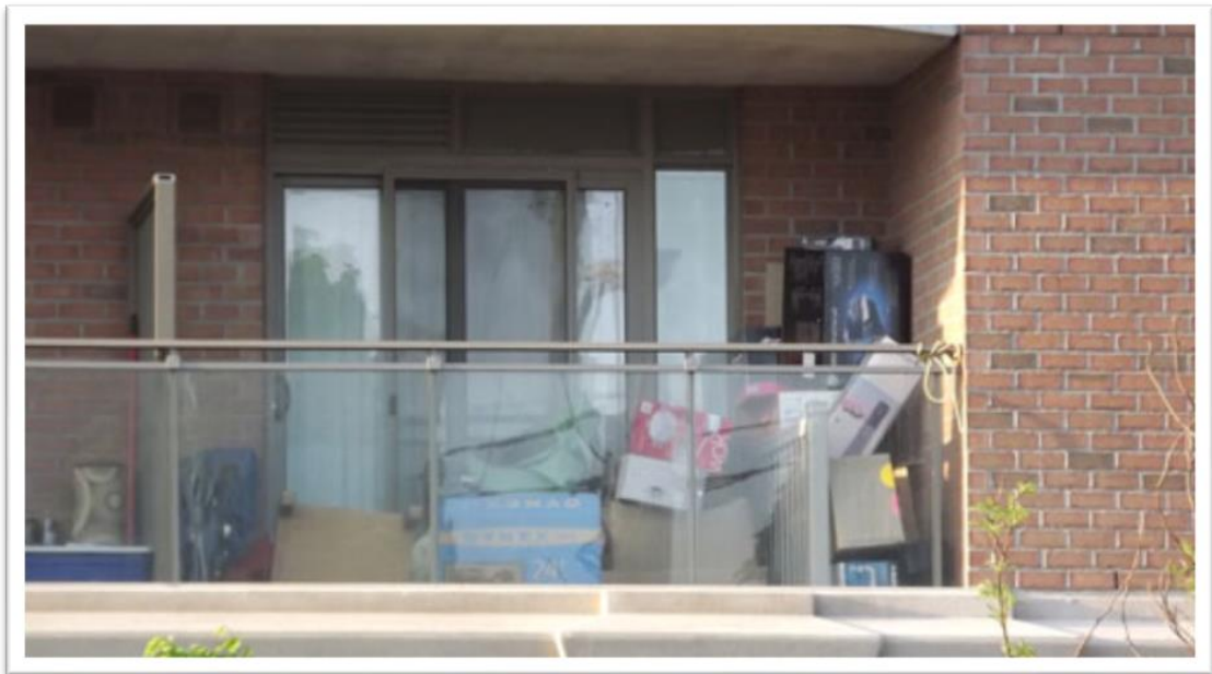
Example of storage on a balcony that should be avoided.
