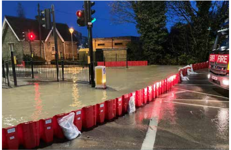
Flood Protection Barriers slot together to divert water away from properties.
