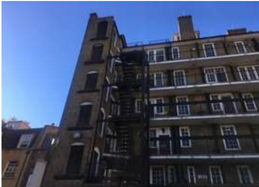
Integrated drill tower
