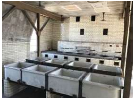
Victorian Washroom (fifth floor)
