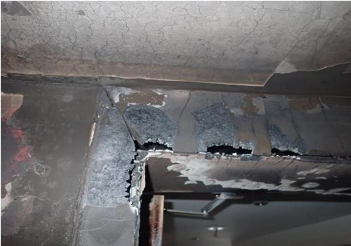
Image showing the timber boxing around the front door frame of flat next to flat of origin
