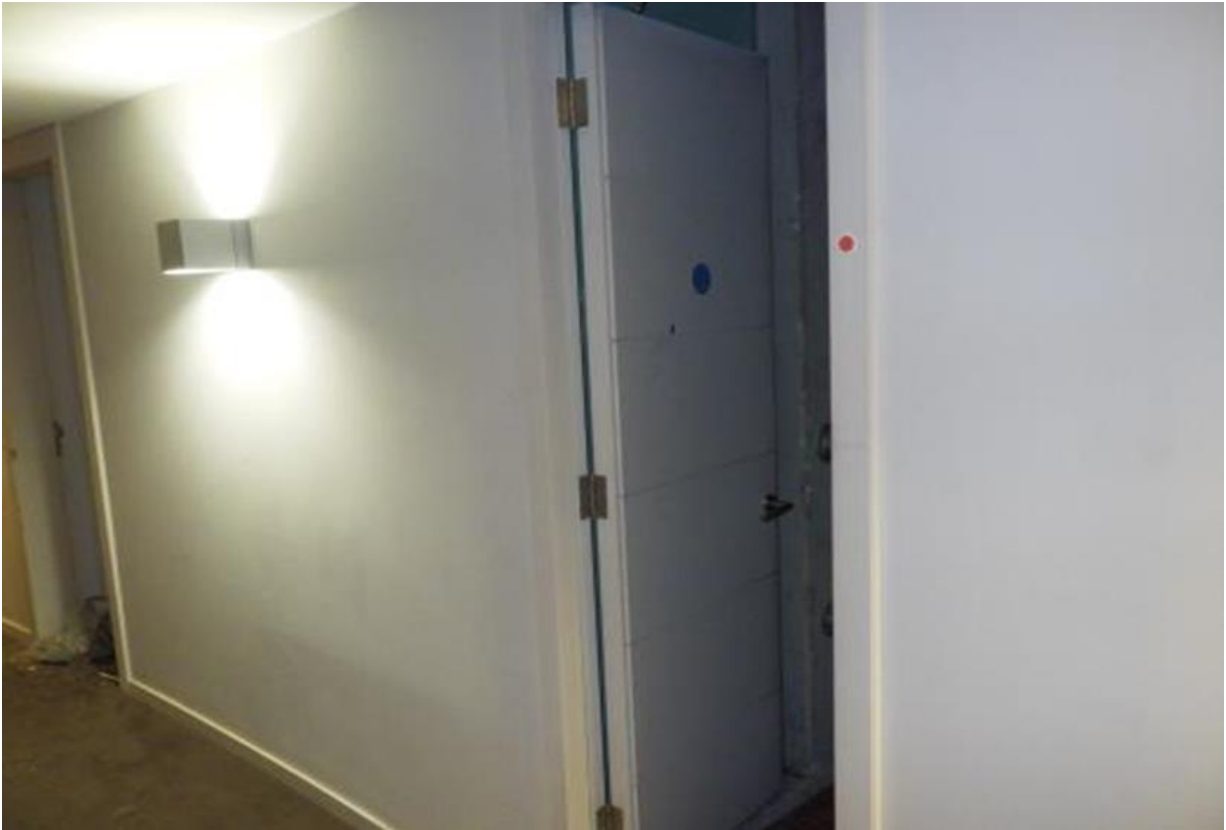
Image showing the AOV door on the 9 th floor
