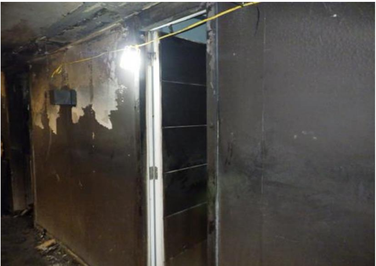
Image showing the AOV door on the 8 th floor
