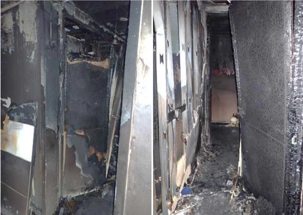
Images showing the front entrance (looking from outside) and hallway (looking from inside) of flat. Note the remains of the door to the left of the doorway
