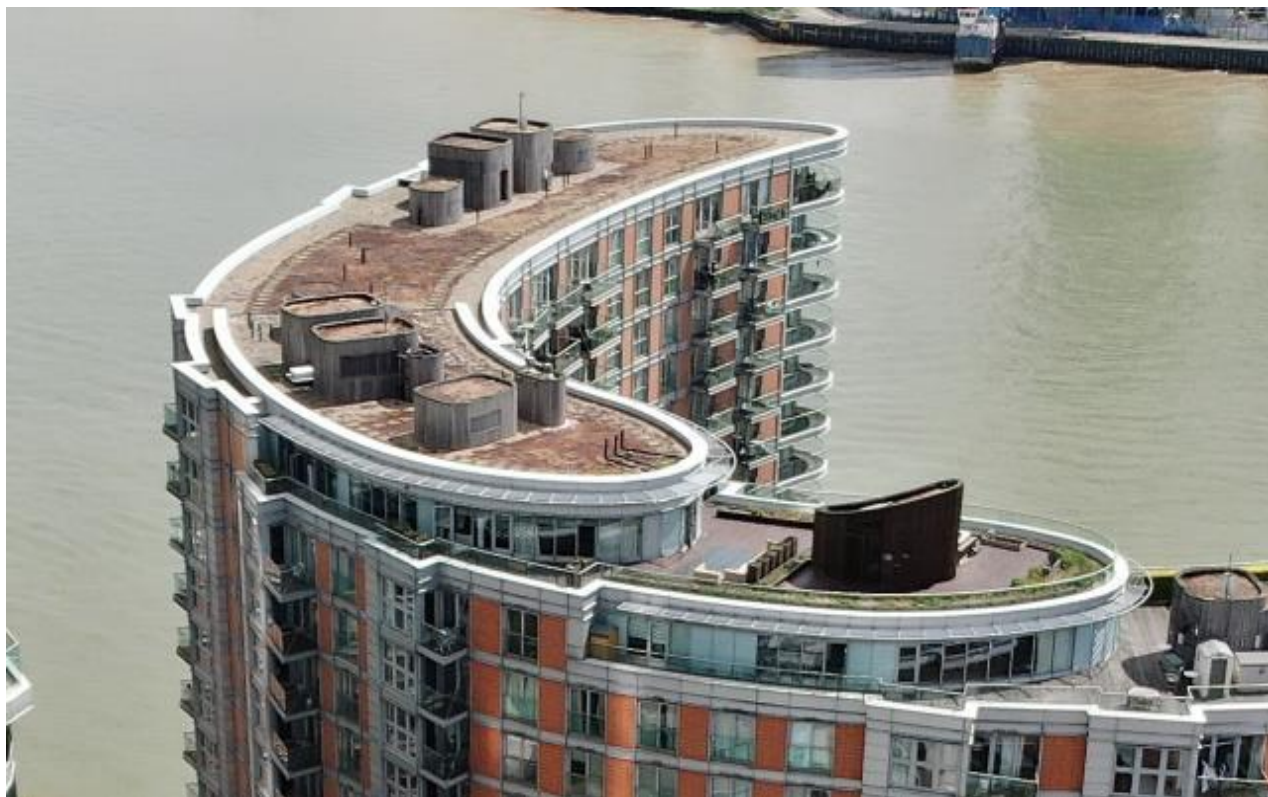
Image showing the roof of New Providence Wharf with AOV vents
