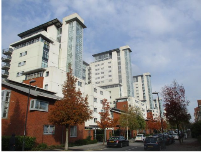
1 – General view of the property.
