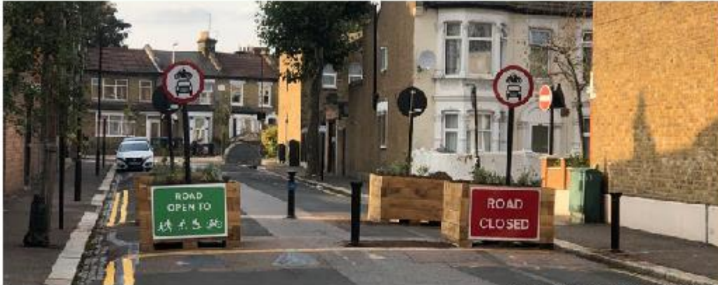
Image of existing modal filter on Blenheim Road
