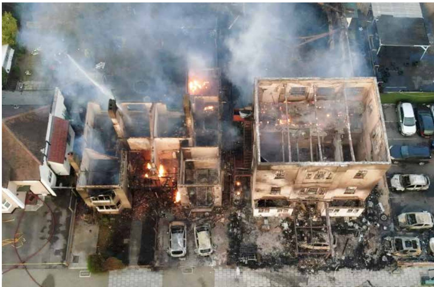
Property damage following the Major Incident in Wennington.
