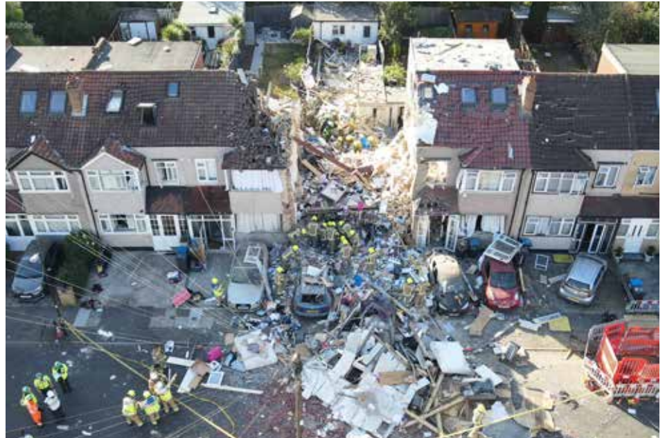
The scene of a gas explosion in South East London where operational discretion was declared.
