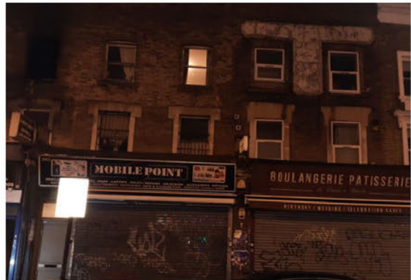
4. Image of the neighbouring property that require a fire safety inspection
