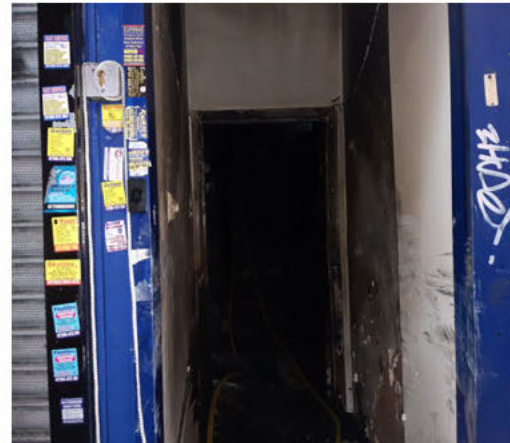
2. Image of entrance to the flats from the pavement
