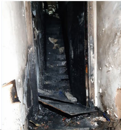
3. Image of the entrance hall and stairs to the first floor
