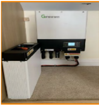
Figure 1 Small scale domestic BESS
